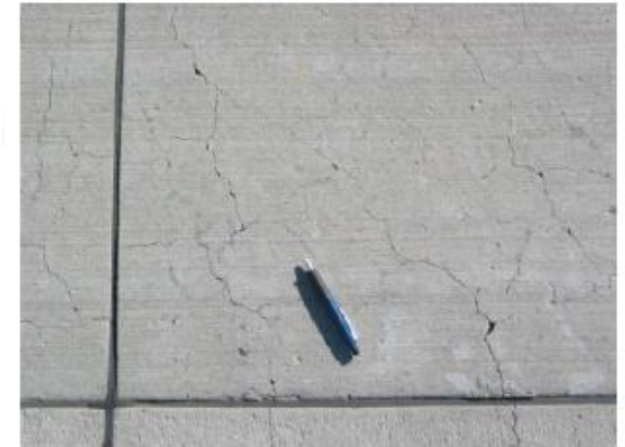
FIG. X2.75 Medium-Severity ASR
