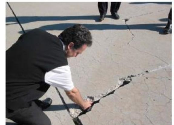
FIG. X2.76 High-Severity ASR
