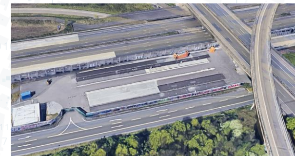
Полигон Federal Highway Research Institute (BASt), Германия
